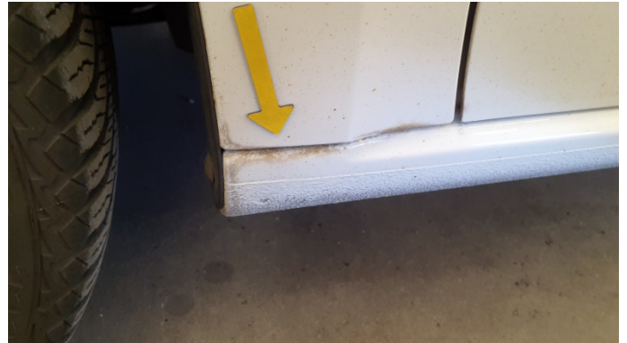
4. Schweller - Links Rost -
